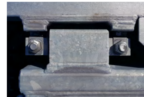
The torsion coupling provides movement in all directions
