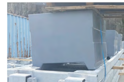
Pontoon during assembly
