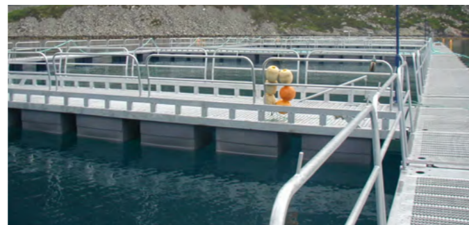
Sections reinforced for forklift driving
